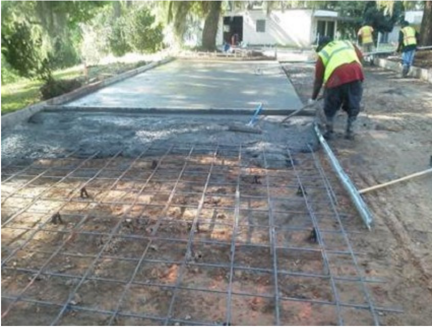
First and second slab poured, third section being worked.
