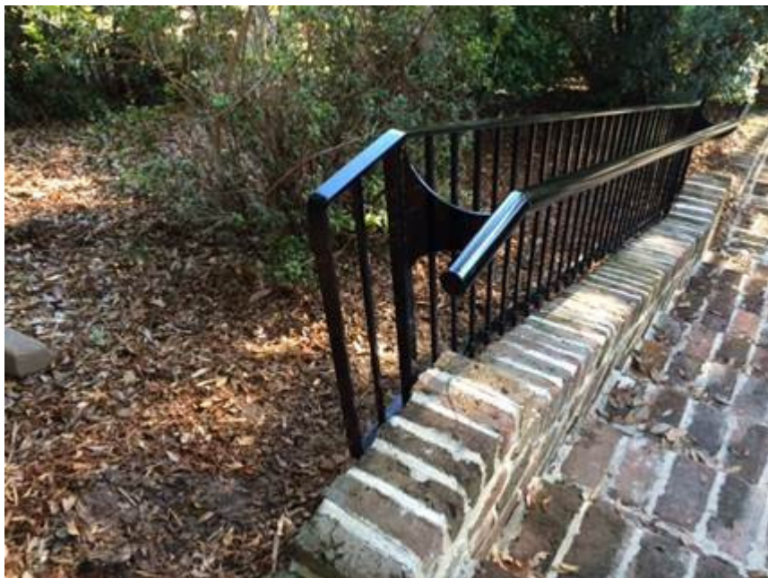
Section of railing at Luce
