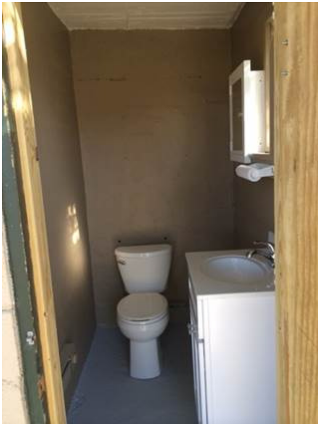
Renovated Breakroom bathroom
