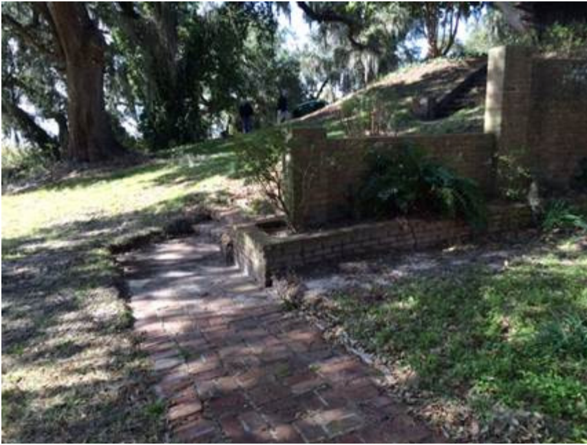
Mystery excavation of brick walkway from Dorm to steps
