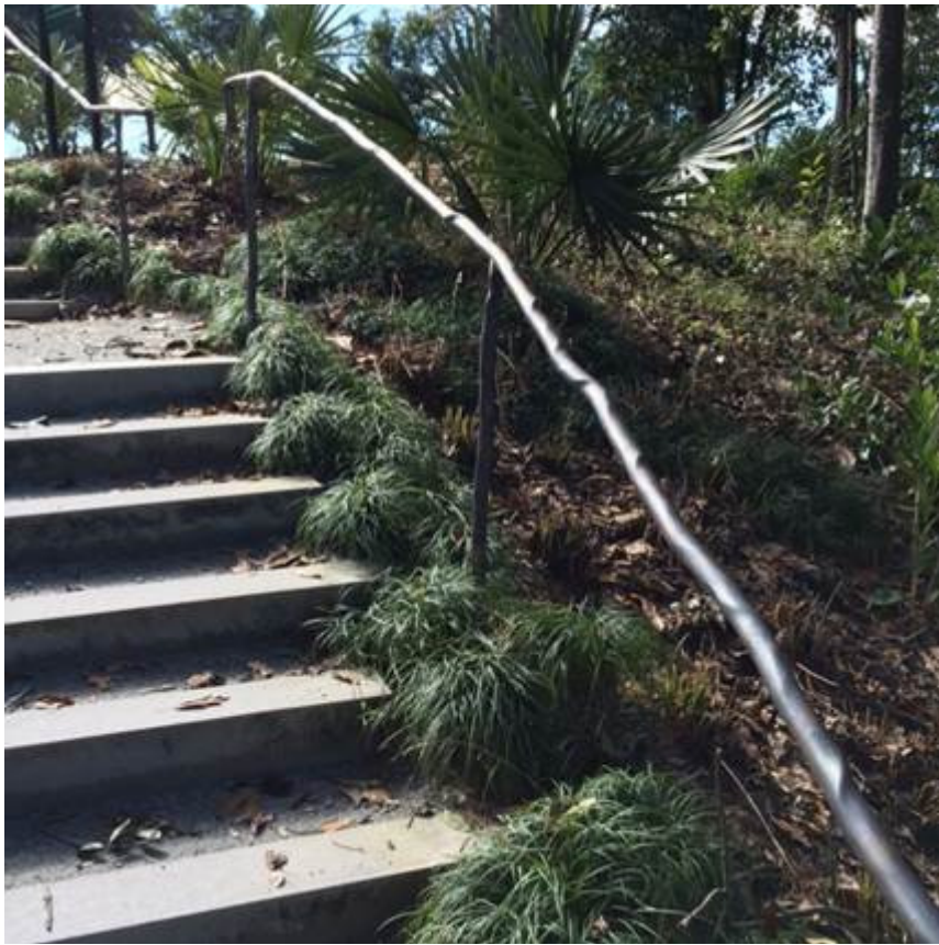
Steps going down
