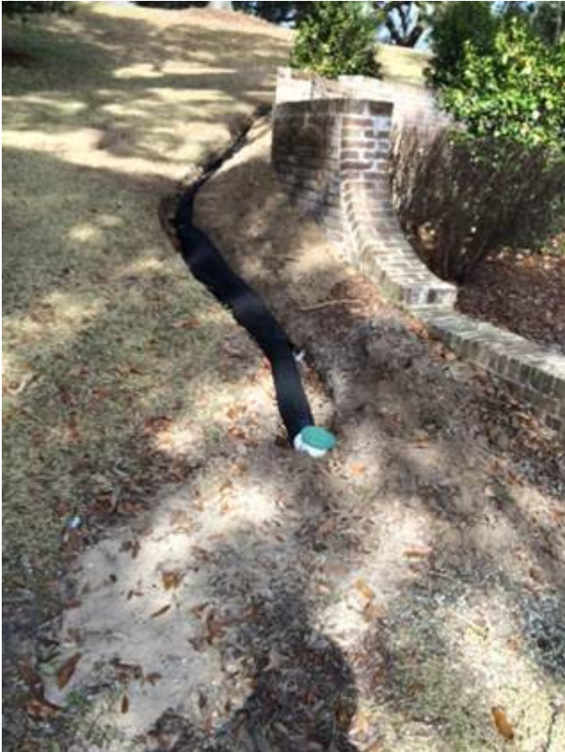
Drainage project in progress
