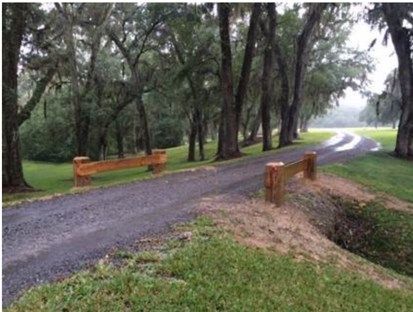
New Culvert Protectors
