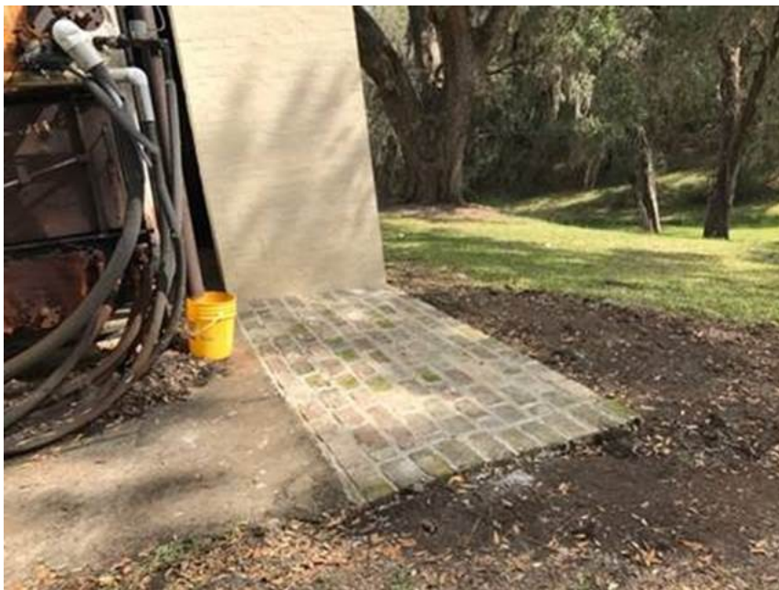
New bricked area at Boiler
