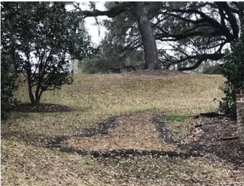
Sodding where the drainage problem has washed away the grass
