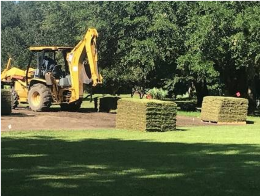
Sodding Columbarium in progress
