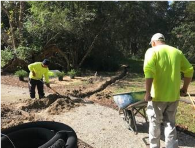
Trenching the water line to the soaker system
